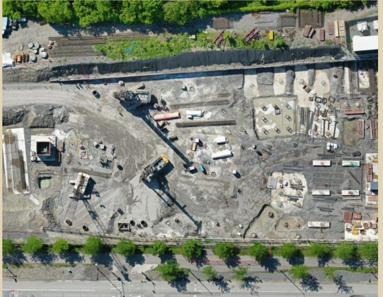
Drilled caissons bridging CSST
